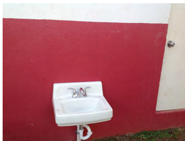
New sink installed to facilitate frequent handwashing
